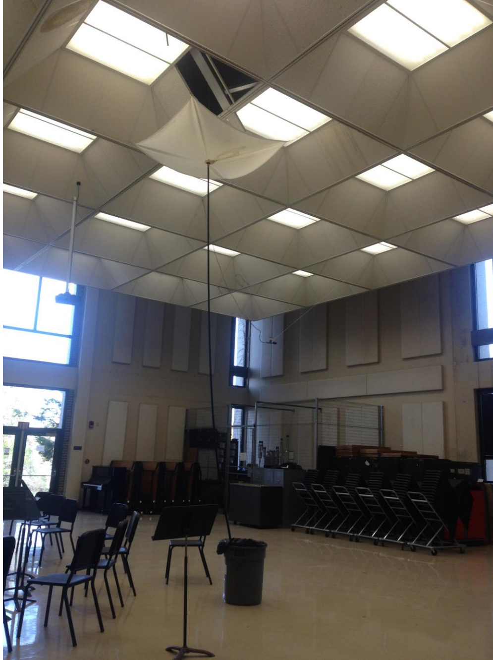
Major Roof Deterioration/Water infiltration during rainy weather. Requires Replacement
