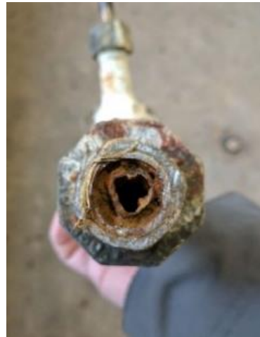
Internal pipe damage
