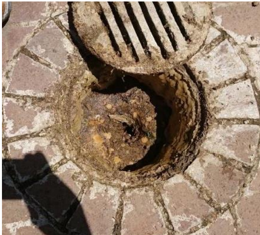
Internal drain damage
