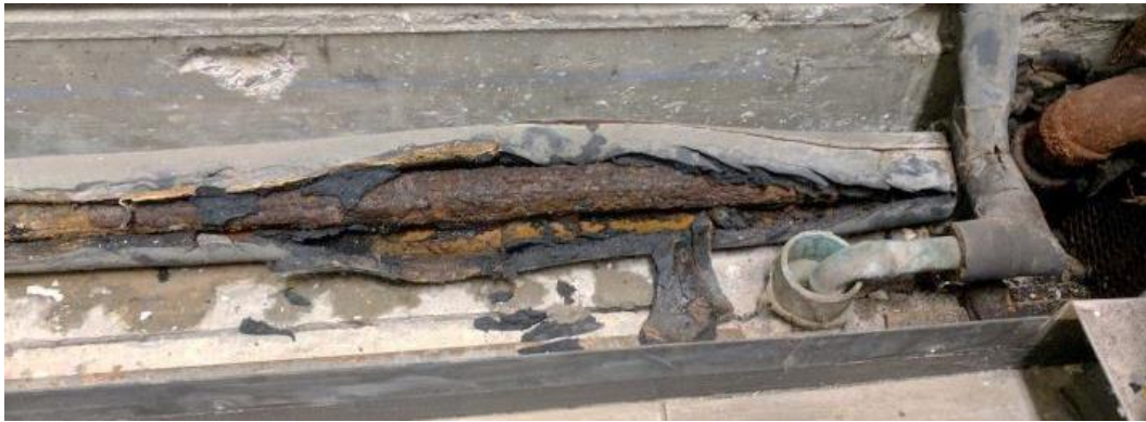
Pipe casing damage
