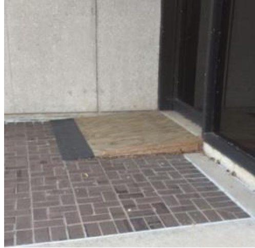
Temporary wooden ramp
