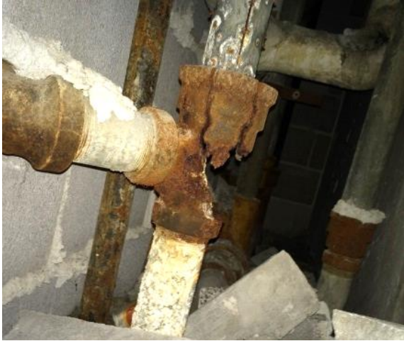
Completely rotted pipe
