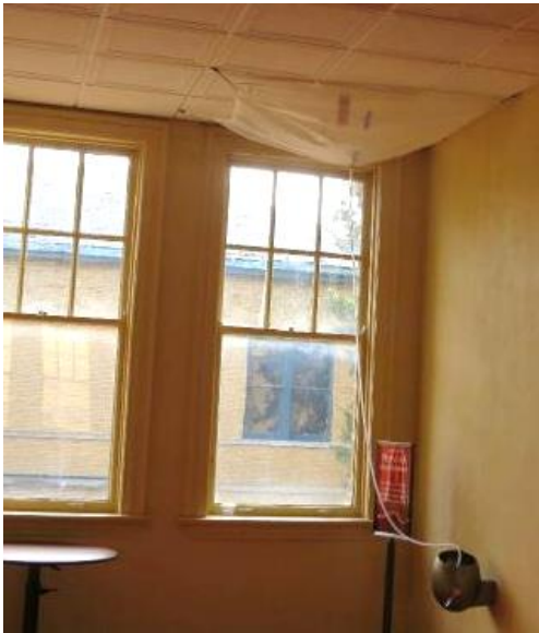
Ceiling leak (with improvised drainage system)
